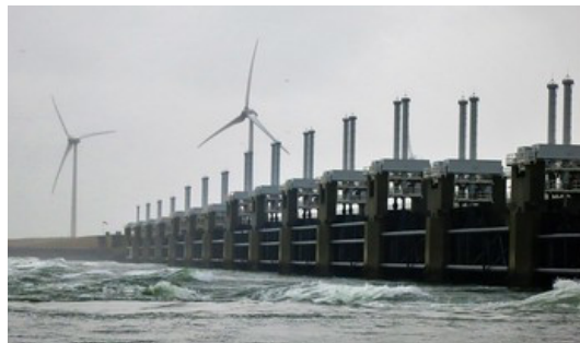
The Delta Works in the Netherlands, consisting of 13 sections, together form the largest flood protection system in the world. (© Mirko Tobias Schäfer )
